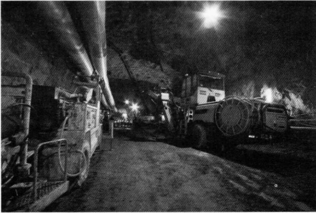
Machinery inside the tunnel. Photo Lars Hansson
